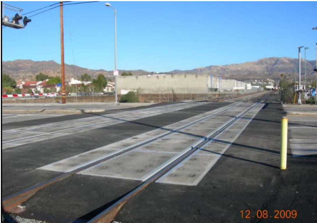
SCRRRA track work at Lassen St. at-grade rail crossing
