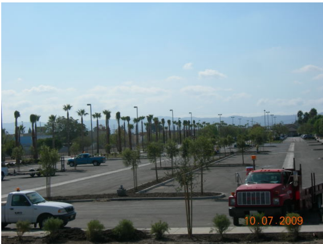
Completed construction of North Parking Lot at Chatsworth Station.
