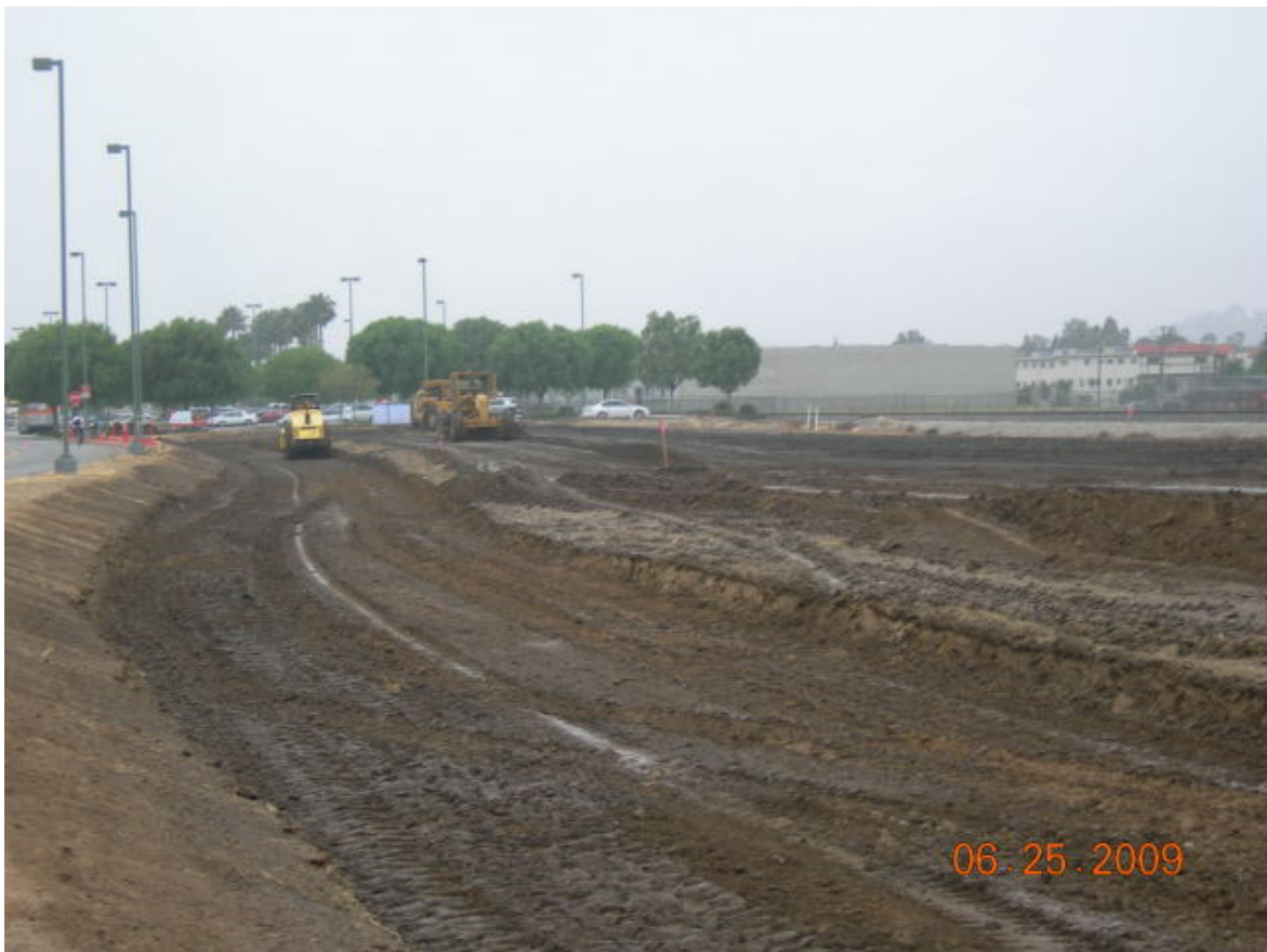
Site grading at Contract C0941 North Parking Lot (Chatsworth Station).
