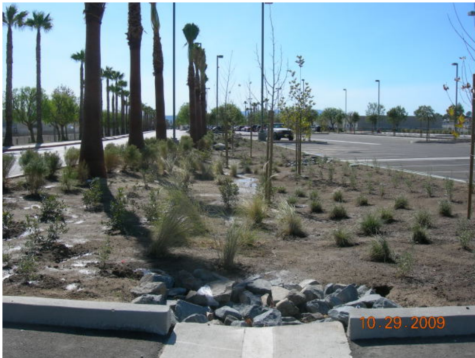
Chatsworth Metrolink Station Site - Bio-cell feature within North Parking Lot.
