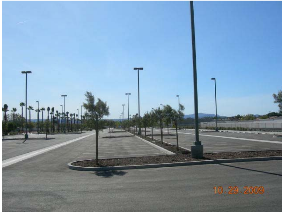
Chatsworth Metrolink Station Site - completed North Parking Lot.
