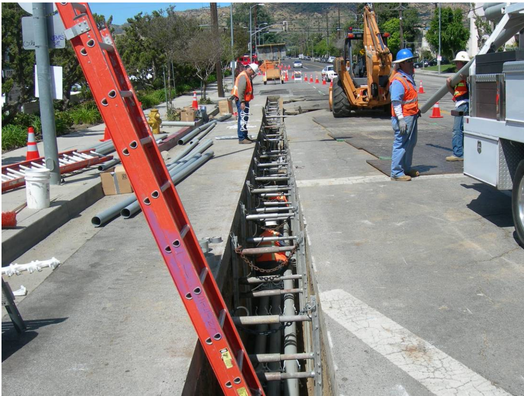
Design Builder continues construction of underground utility work on Lassen Street.
