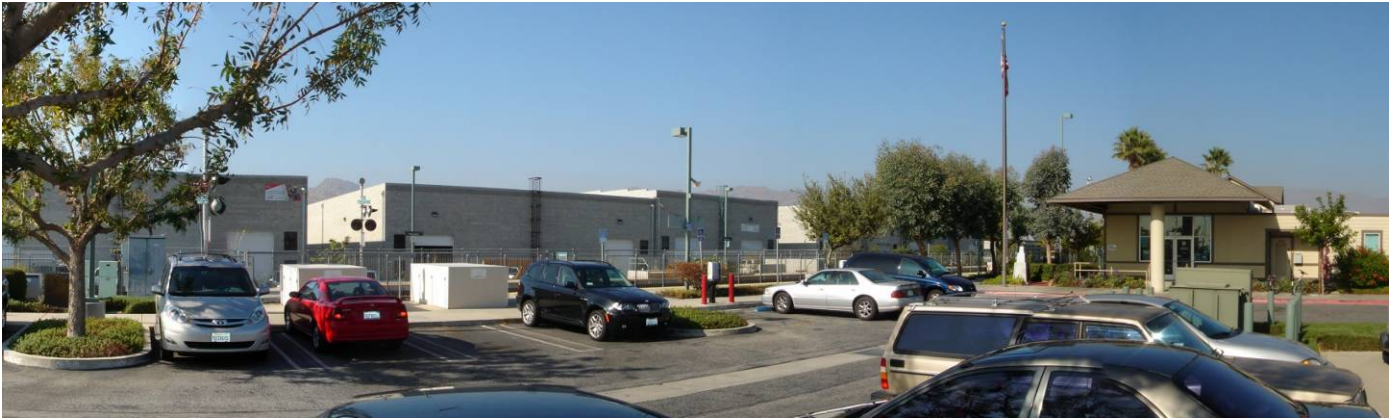
Current view Chatsworth Station.
