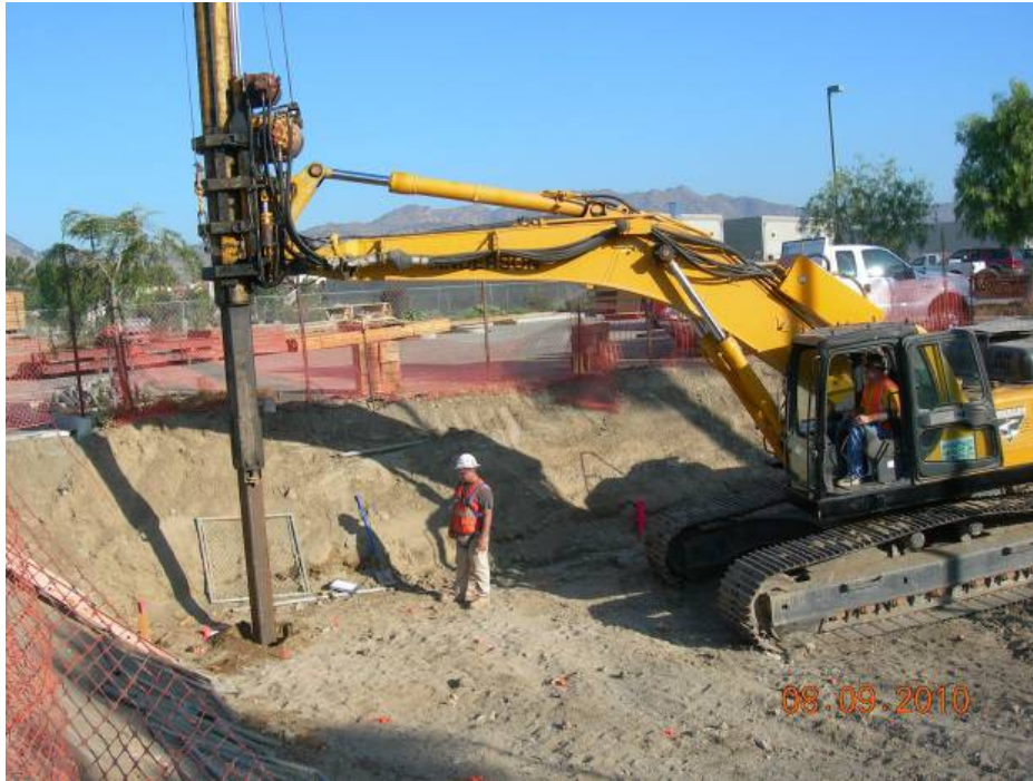
Drilling for pile foundations – Lassen Bridge.
