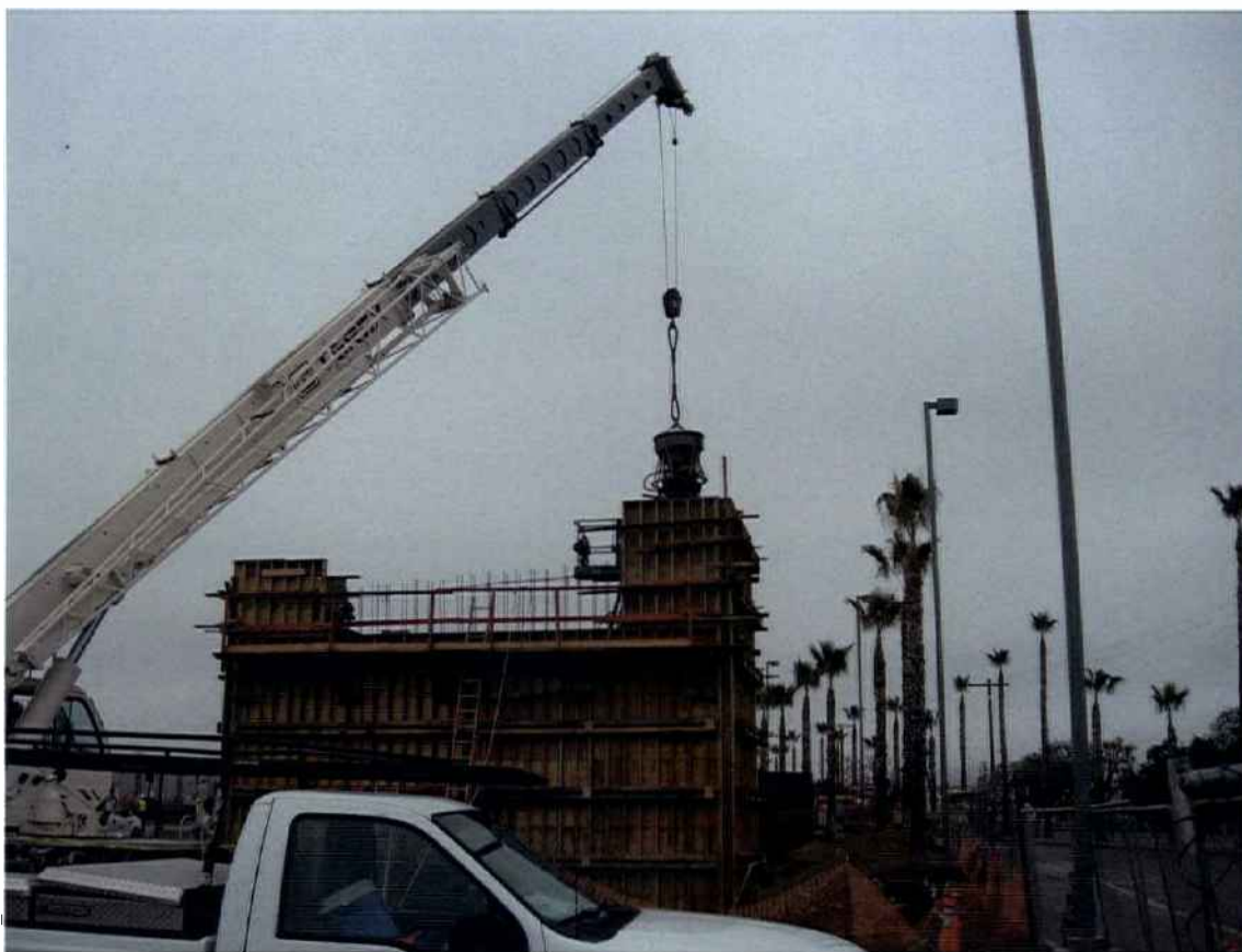
C0943 Design Build Contractor placing abutment 4 shear key wall.
