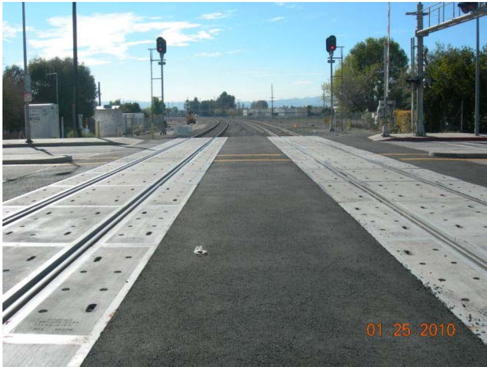
SCRRRA replaced track at Lassen rail crossing.
