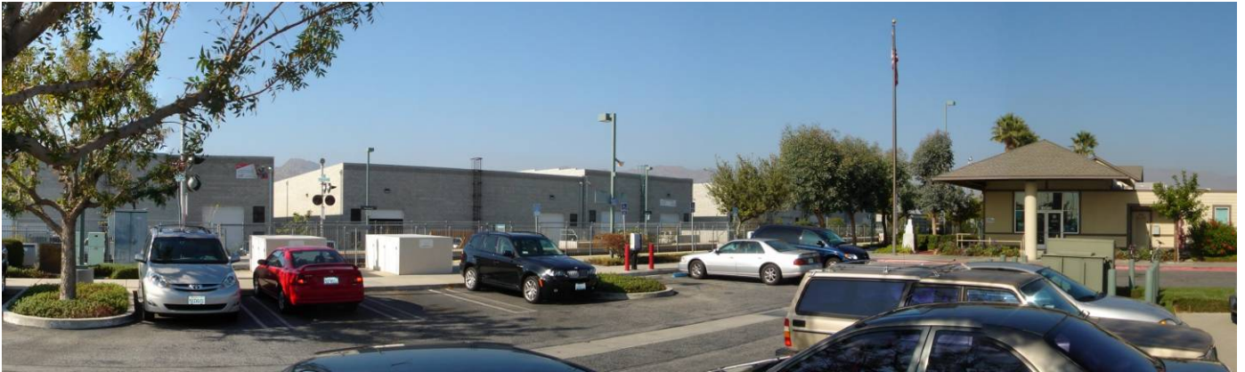
Current view Chatsworth Station.
