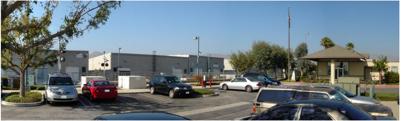
Current view Chatsworth Station.
