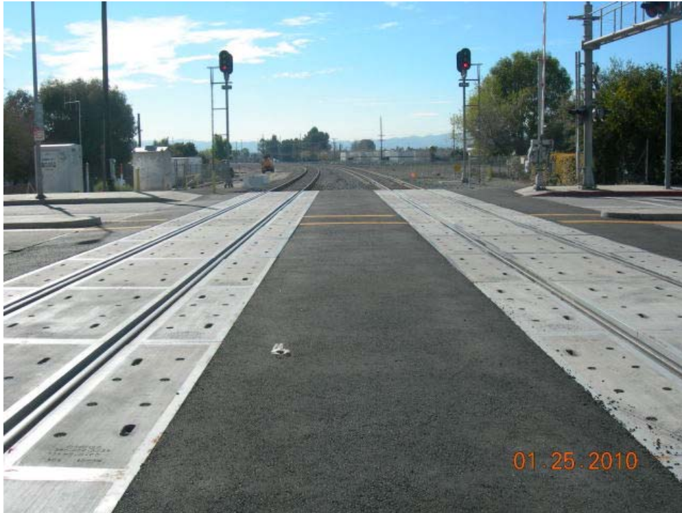
SCRRRA replaced track at Lassen rail crossing.
