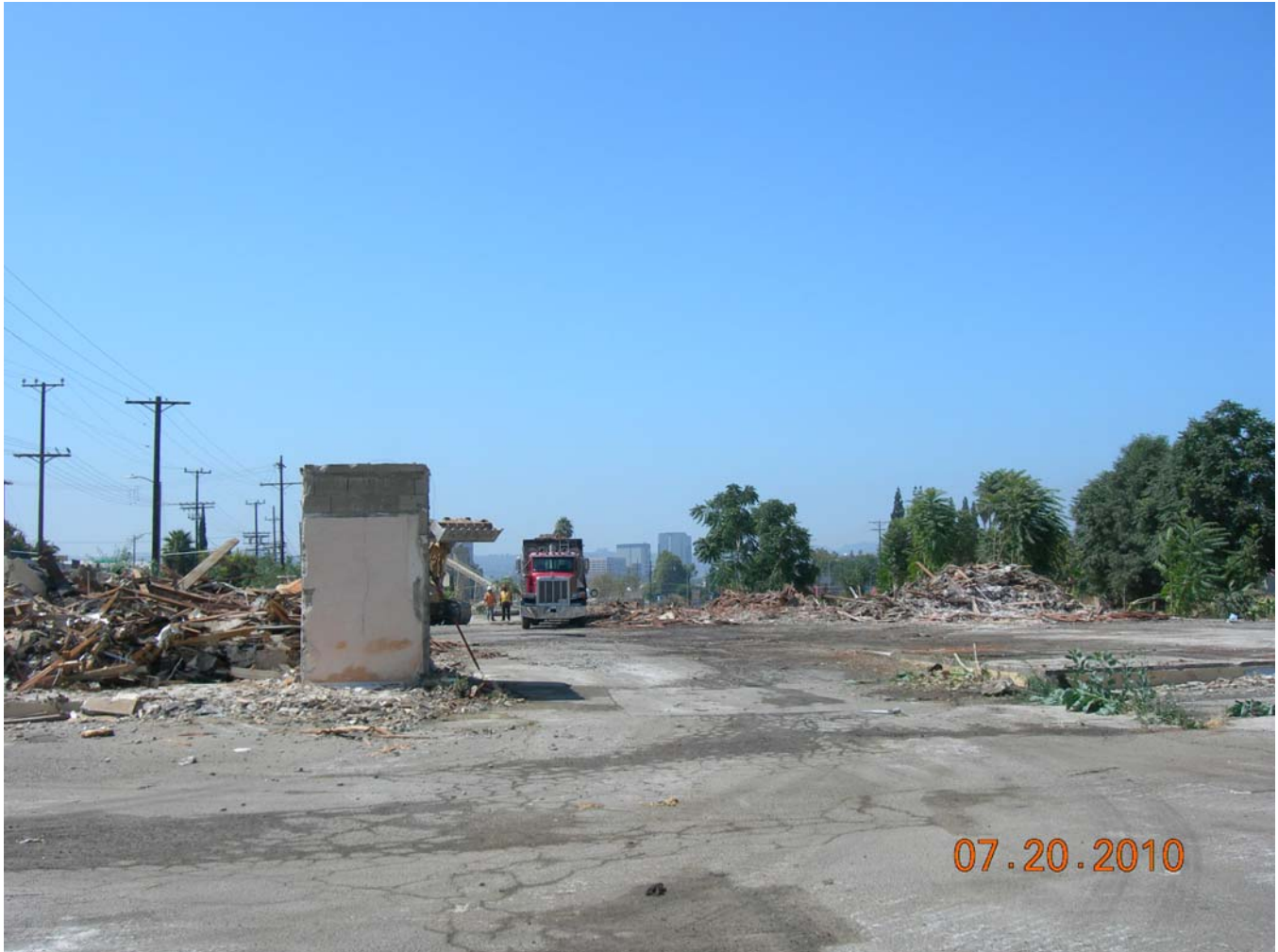
Right-of-way demolition at Sherman Way and Canoga Avenue.
