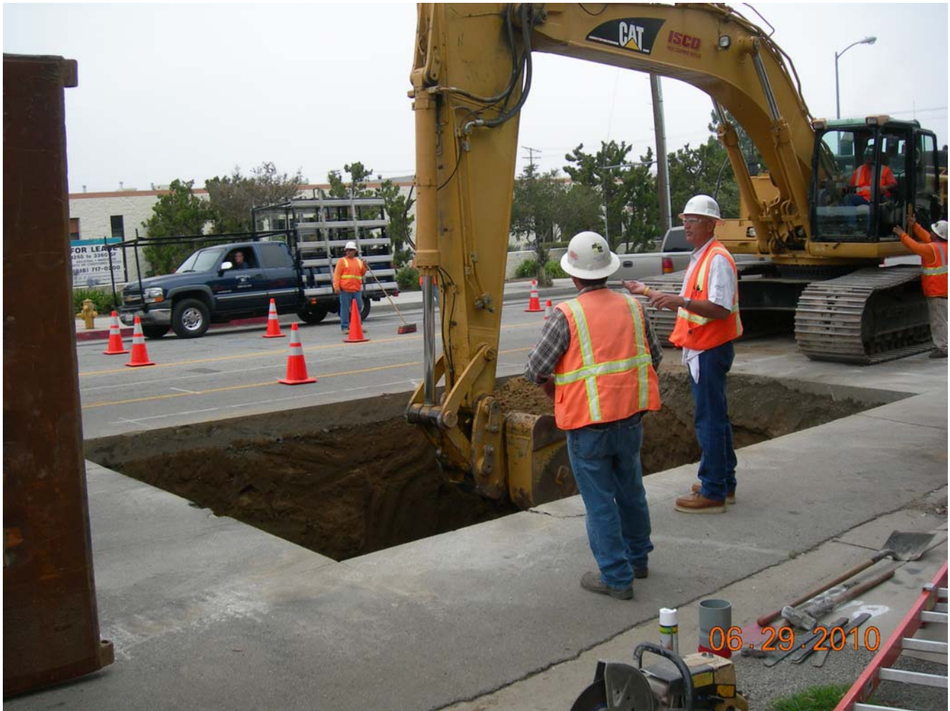
Subcontractor installing vault manhole on Lassen Street.
