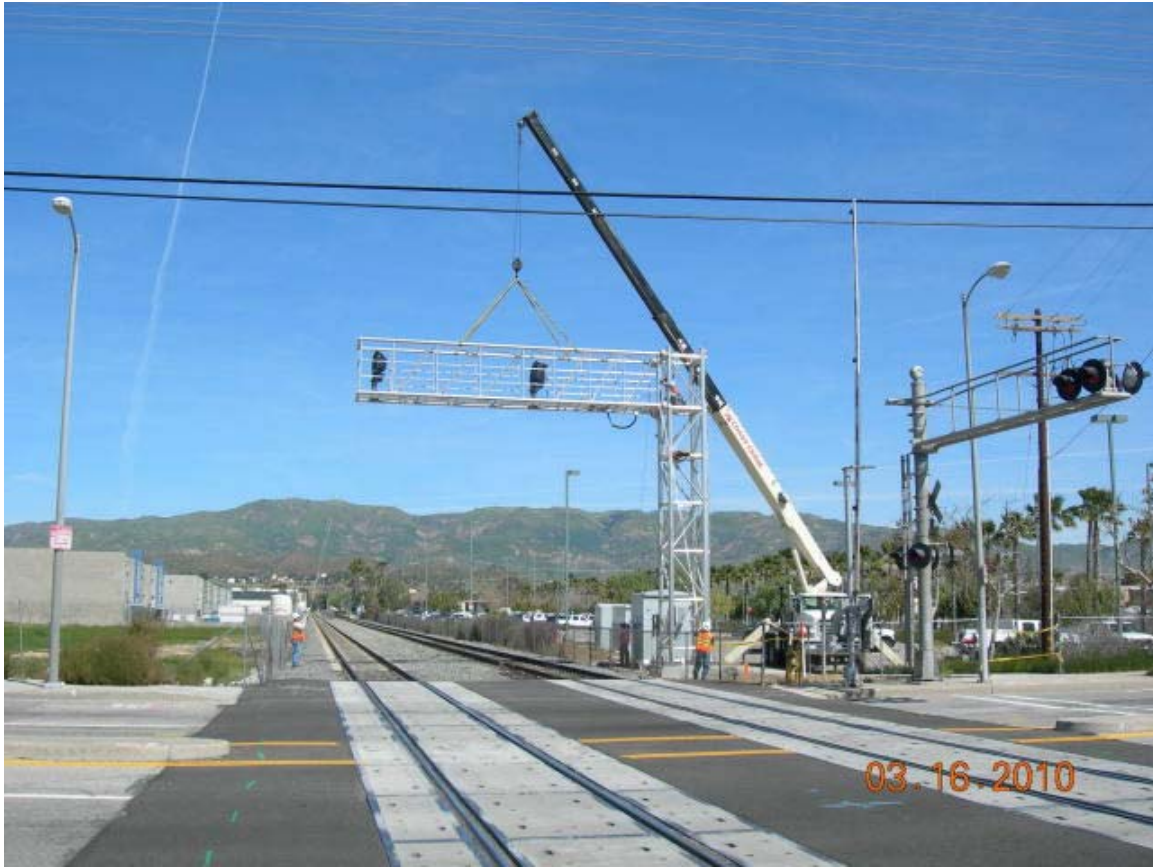
New rail signal work by Metrolink.
