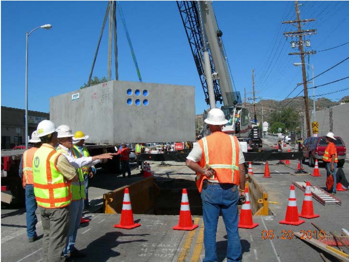
Placing underground vault on Lassen Street.
