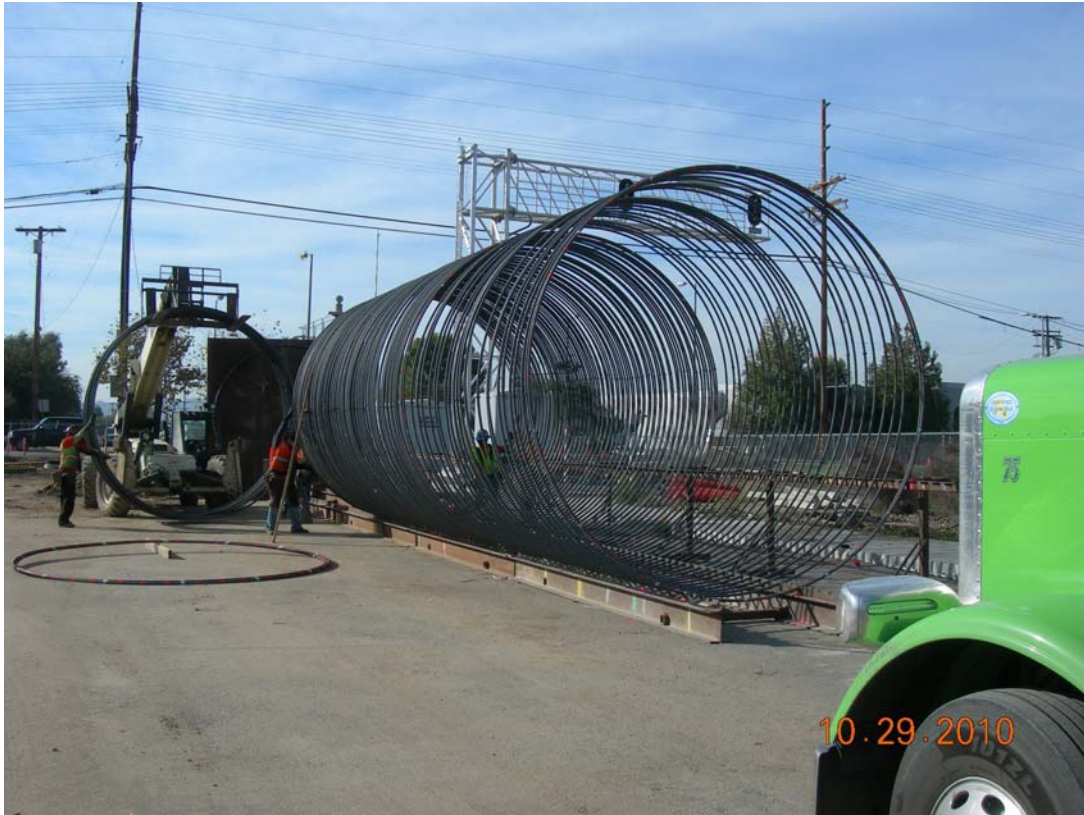
Preparing rebar cage for Lassen Bridge bent # 3.
