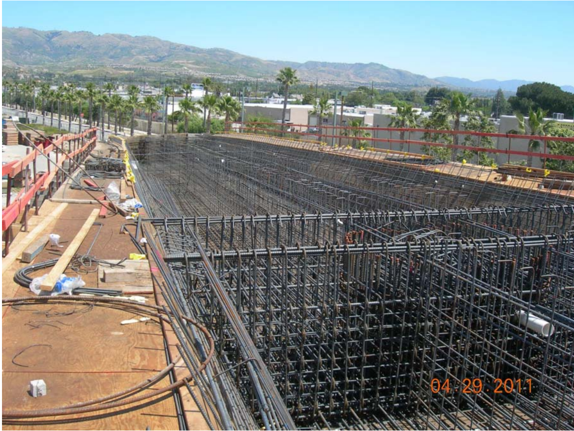
C0943 Design Build Contractor installing reinforcing steel for Lassen Street Bridge.
