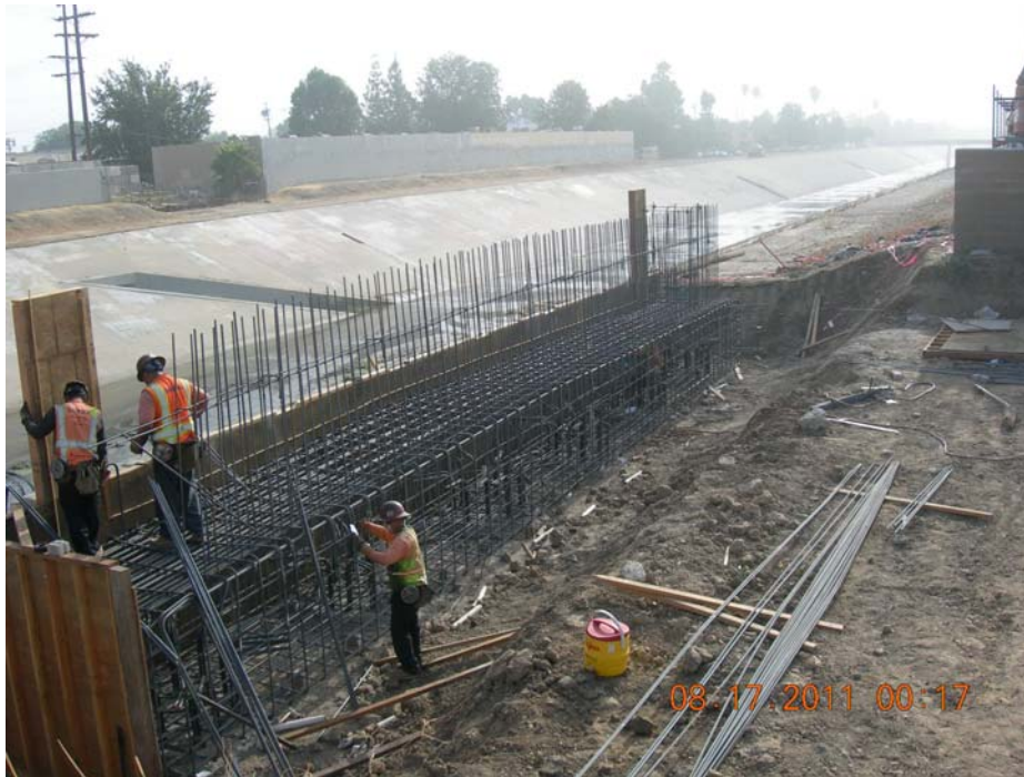
C0943 Design Build Contractor working on new Los Angeles River Bridge.
