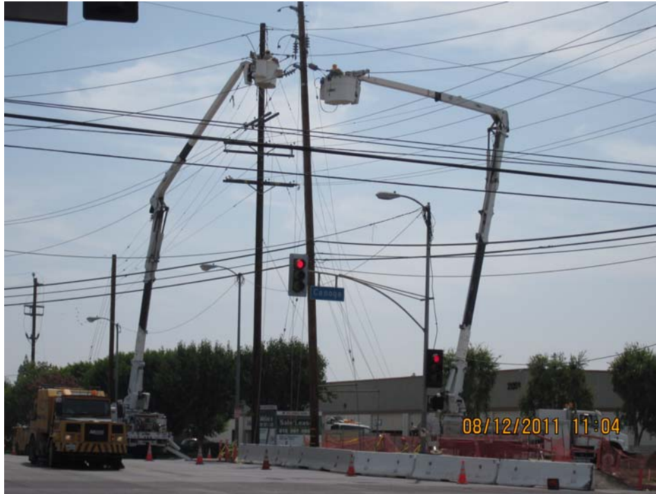
DWP work at intersections.
