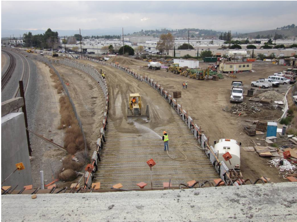
Looking south on top of Lassen Bridge.
