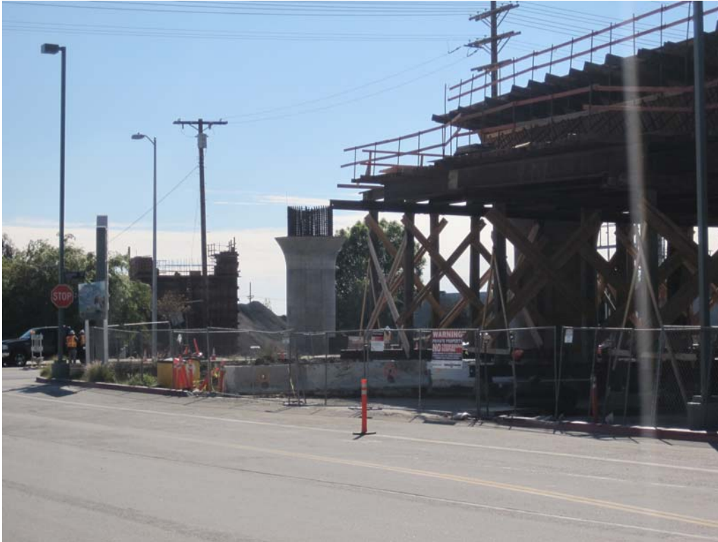
C0943 Design Build Contractor continues installing falsework for the Lassen Bridge.
