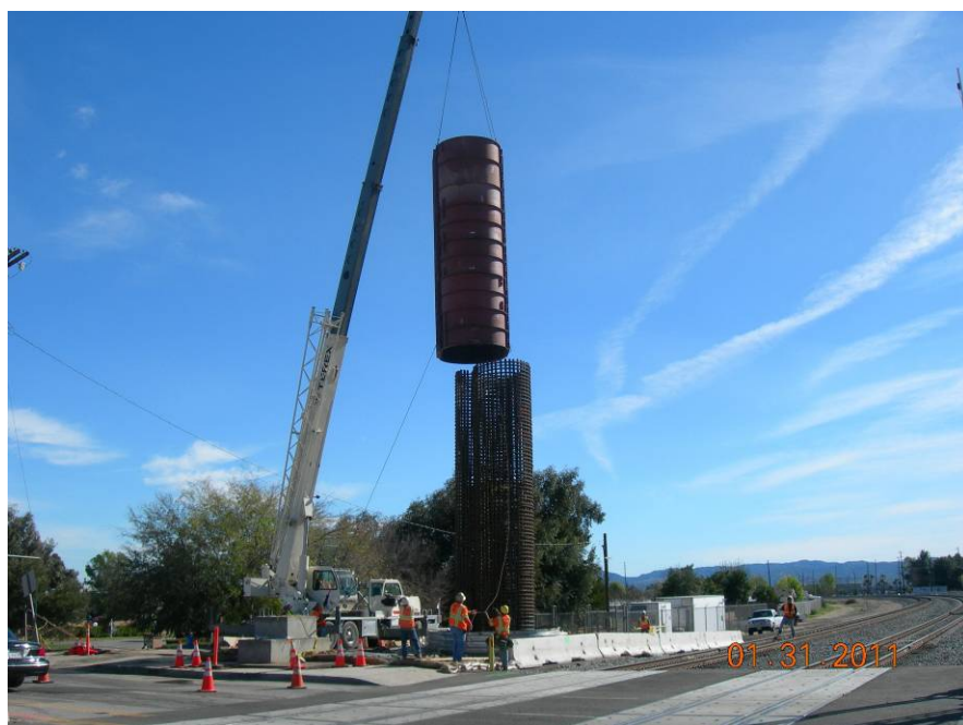
C0943 Design Build Contractor forming bent # 2 column for the Lassen bridge.
