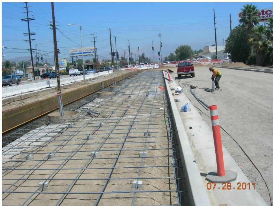
C0943 Design Build Contractor installing reinforcing steel at Roscoe south platform.
