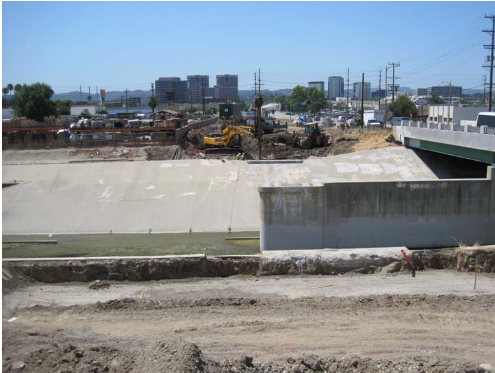
C0943 Design Build Contractor works on new Los Angeles River Bridge.
