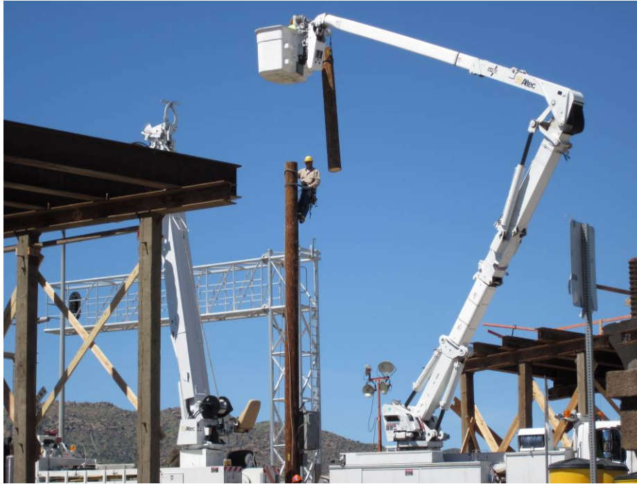
DWP removing conflicting power pole at Lassen Street Bridge.
