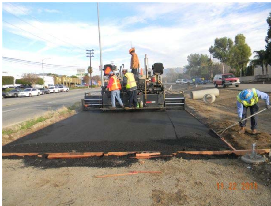
Paving machine on bike path.
