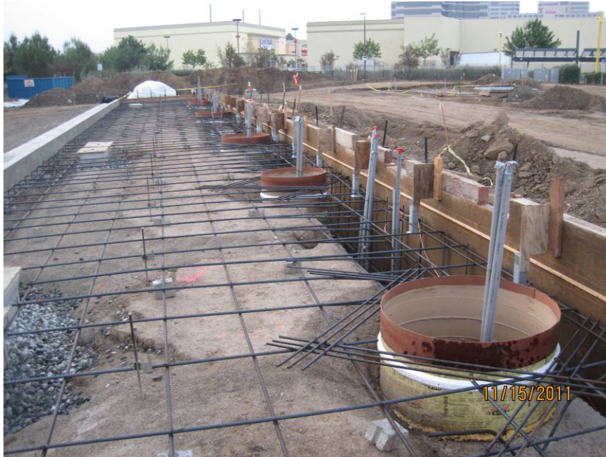
Placing rebar at new Canoga Station south platform.
