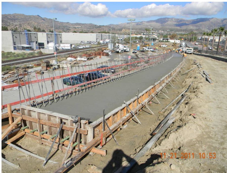
Completed coping slab on MSE Wall #3.
