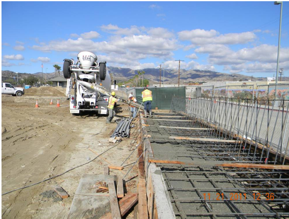
Placing eastside coping slab on MSE Wall #4.
