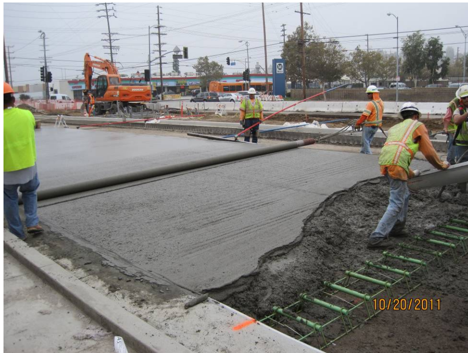
Placing busway pavement at Nordoff.
