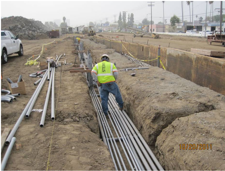
Placing ductbank at Sherman Way Station.
