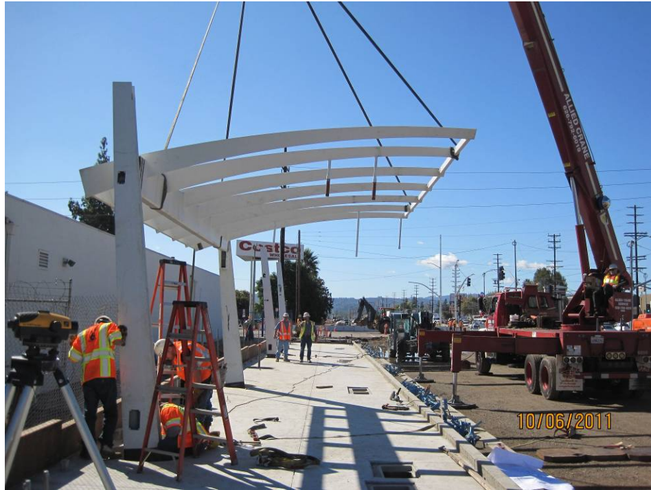
Placing canopy at Roscoe Station.
