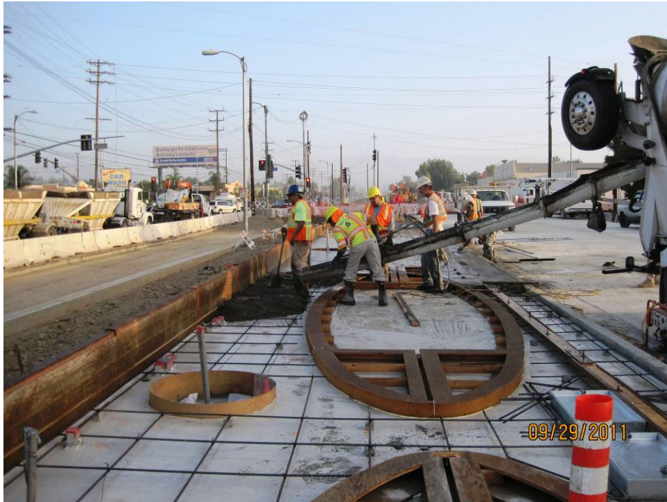
C0943 Design Build Contractor placing topping slab at Roscoe Station.
