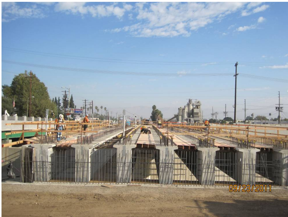
C0943 Design Build Contractor forming LA River Deck.
