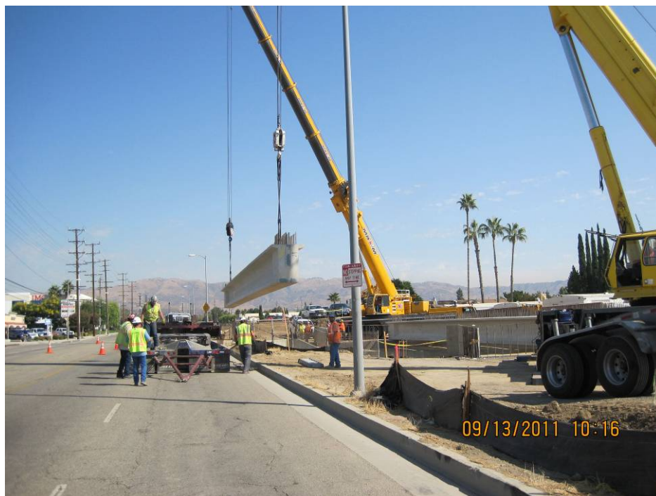
C0943 Design Build Contractor installing girders for Santa Susana Bridge.
