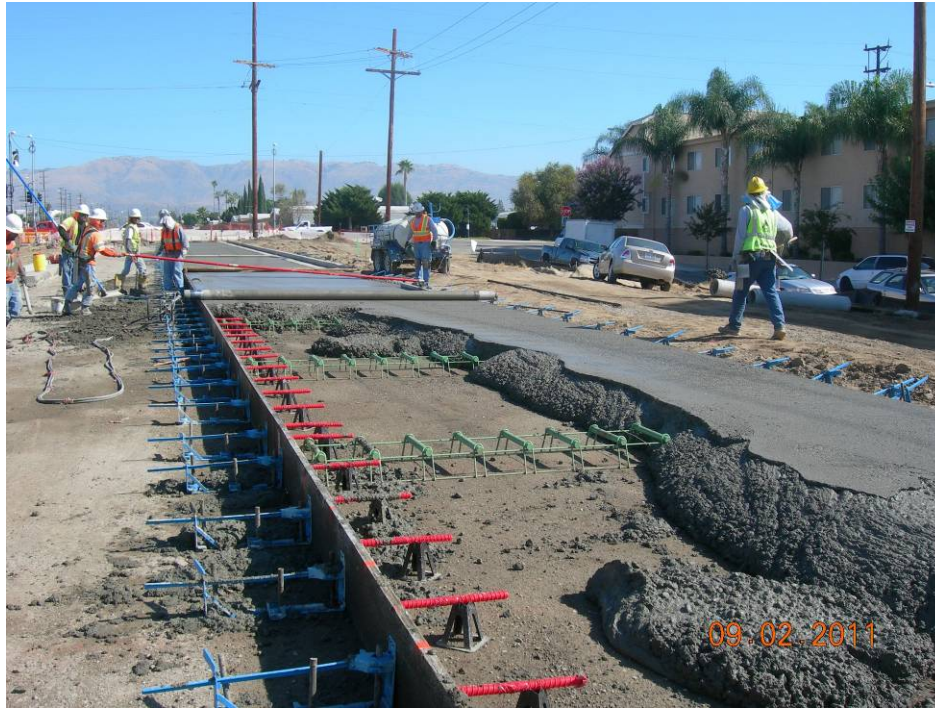
C0943 Design Build Contractor pouring BRT PCC Paving.
