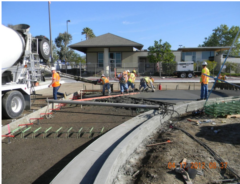
Paving at Chatsworth Station.
