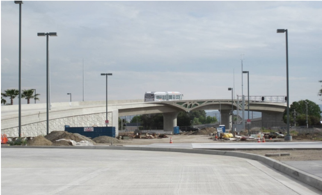
Bus testing over Lassen Bridge.
