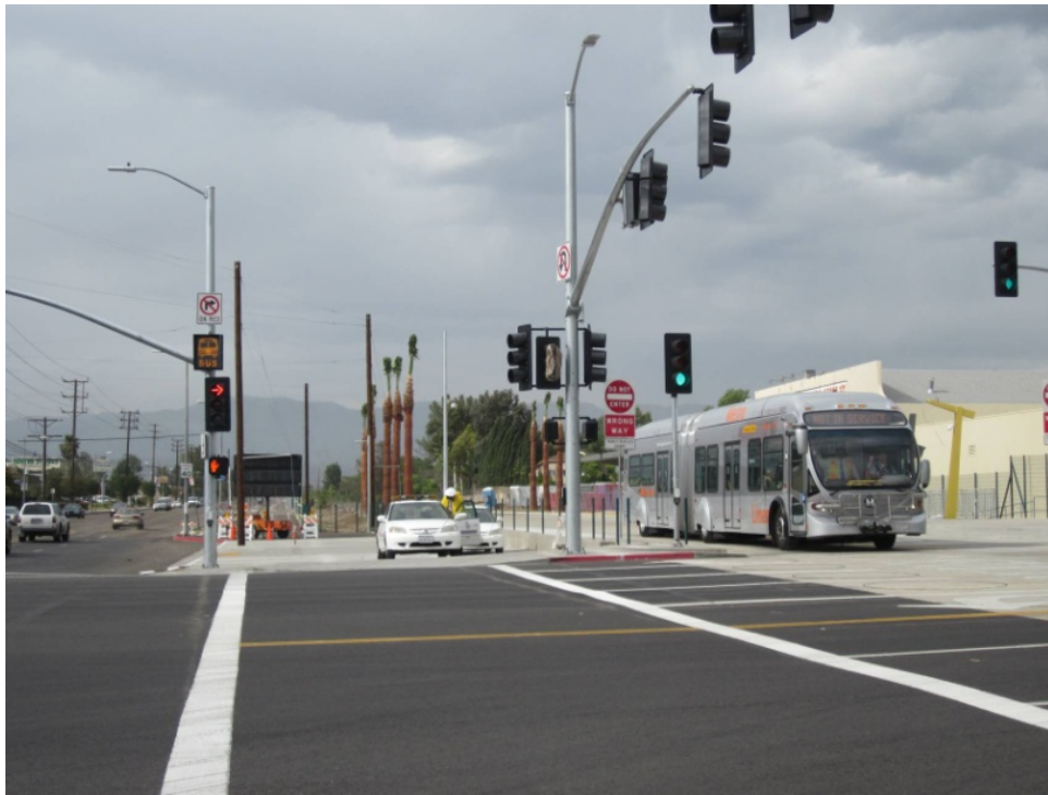
Bus testing on alignment.
