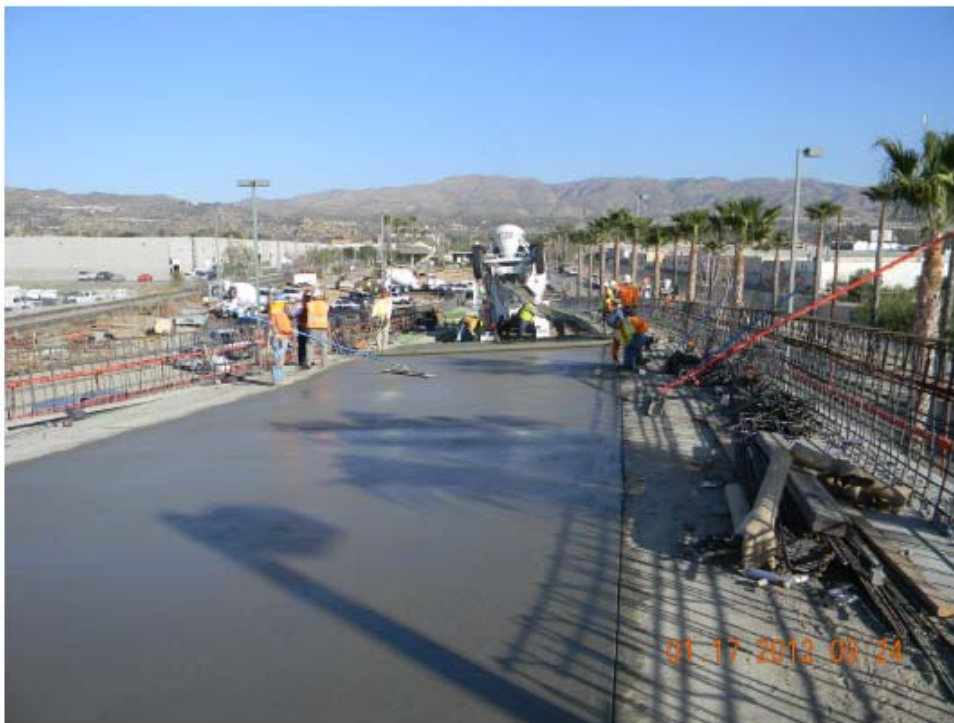
Lassen Bridge paving.
