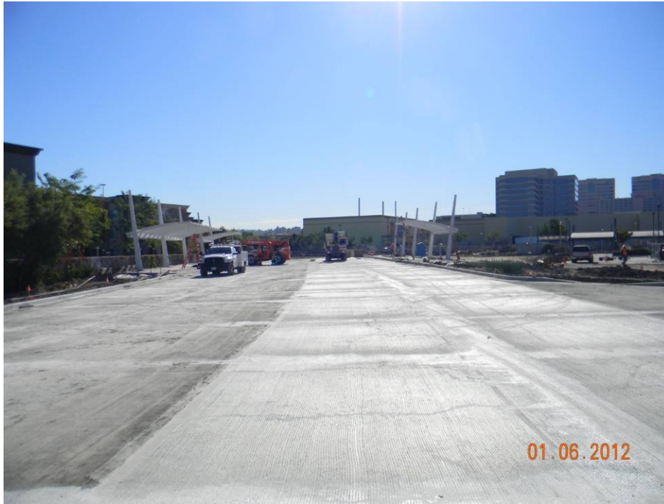
New Canoga Station platforms at interface with existing Metro Orange Line.
