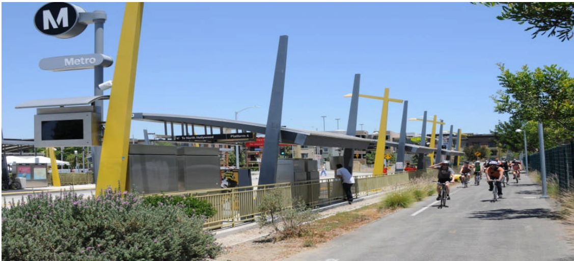
Revenue Service commences on June 30, 2012 – Canoga Station.
