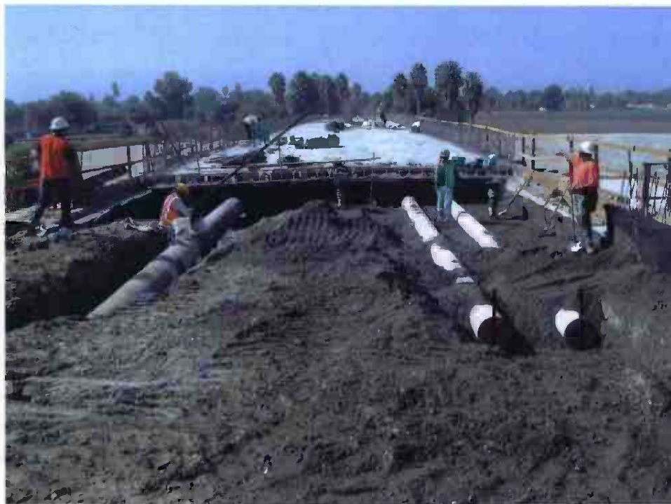
Contract C0676 Los Angeles River Bridge Contractor completed deck placement.
