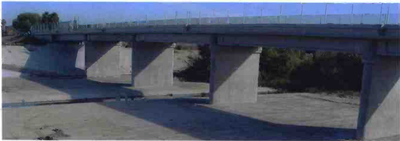
Contract C0676 Los Angeles River Bridge – Completed bridge.
