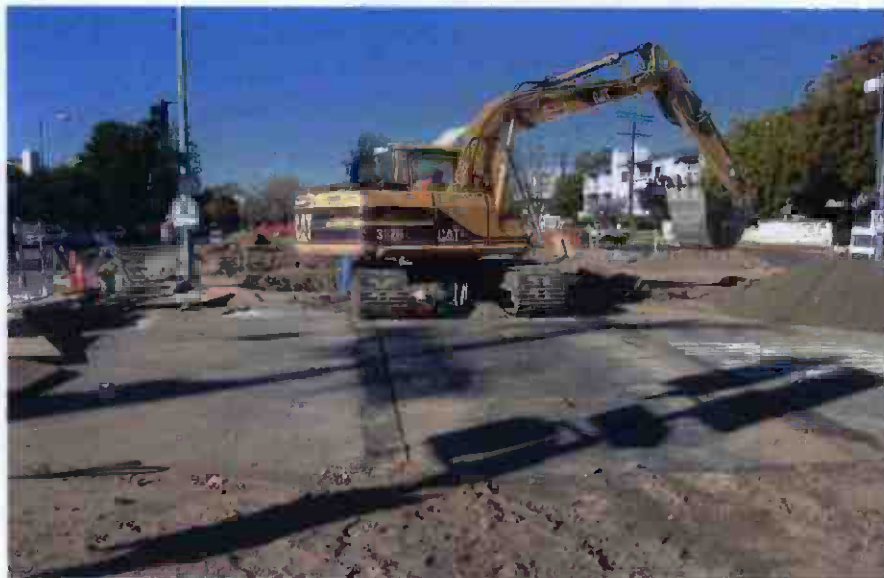
Street closure and storm drain pipe installation at Corteen Avenue.
