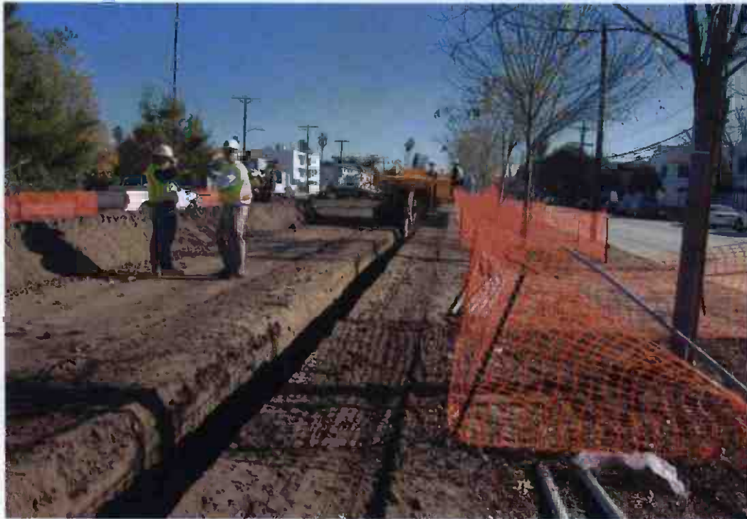
Ductbank installation at Laurel Canyon Blvd. (Eastside).
