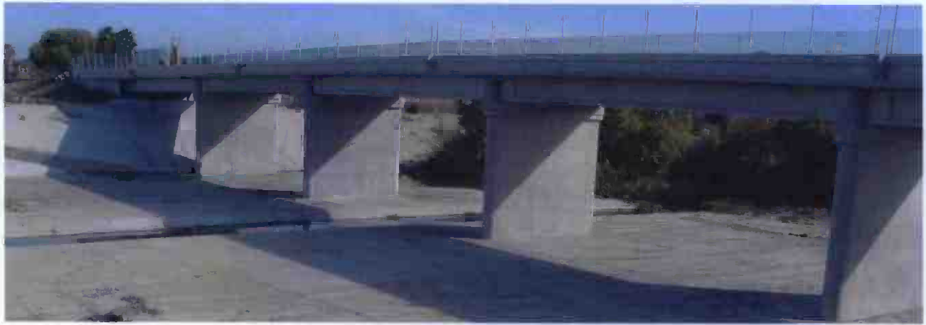
Contract C0676 Los Angeles River Bridge Contractor completed bridge (December 2003).
