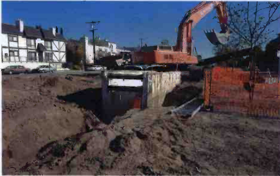
Trench operation for storm drain pipe installation near Laurel Canyon Blvd.
