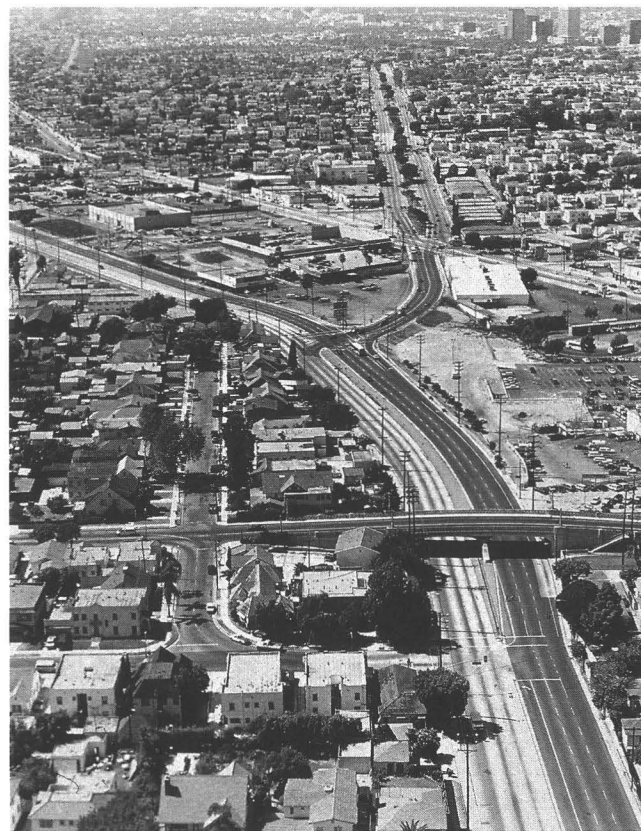
Pico Boulevard-San Vicente Blvd. Aerial photo from Segment 3 Red Line Extension Study
