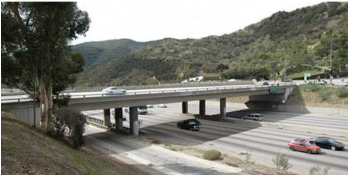
Bridge at Skirball Center Drive over the 405/Metro photo
