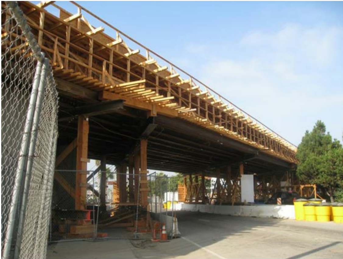
Expo Line construction at Venice and Robertson boulevards.
