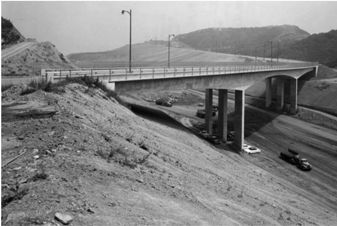
The Mulholland Bridge, completed in 1960, will be demolished and rebuilt. Caltrans photo
