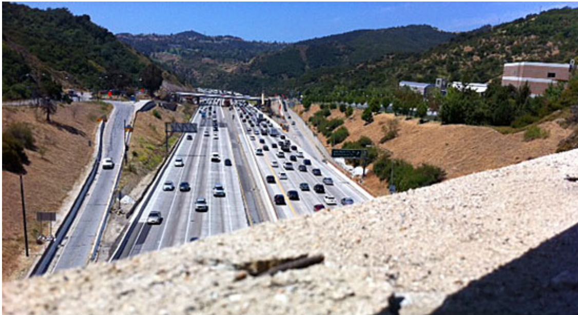
Looking south at the 405 Freeway from the soon-to-be demolished Mulholland Bridge.
