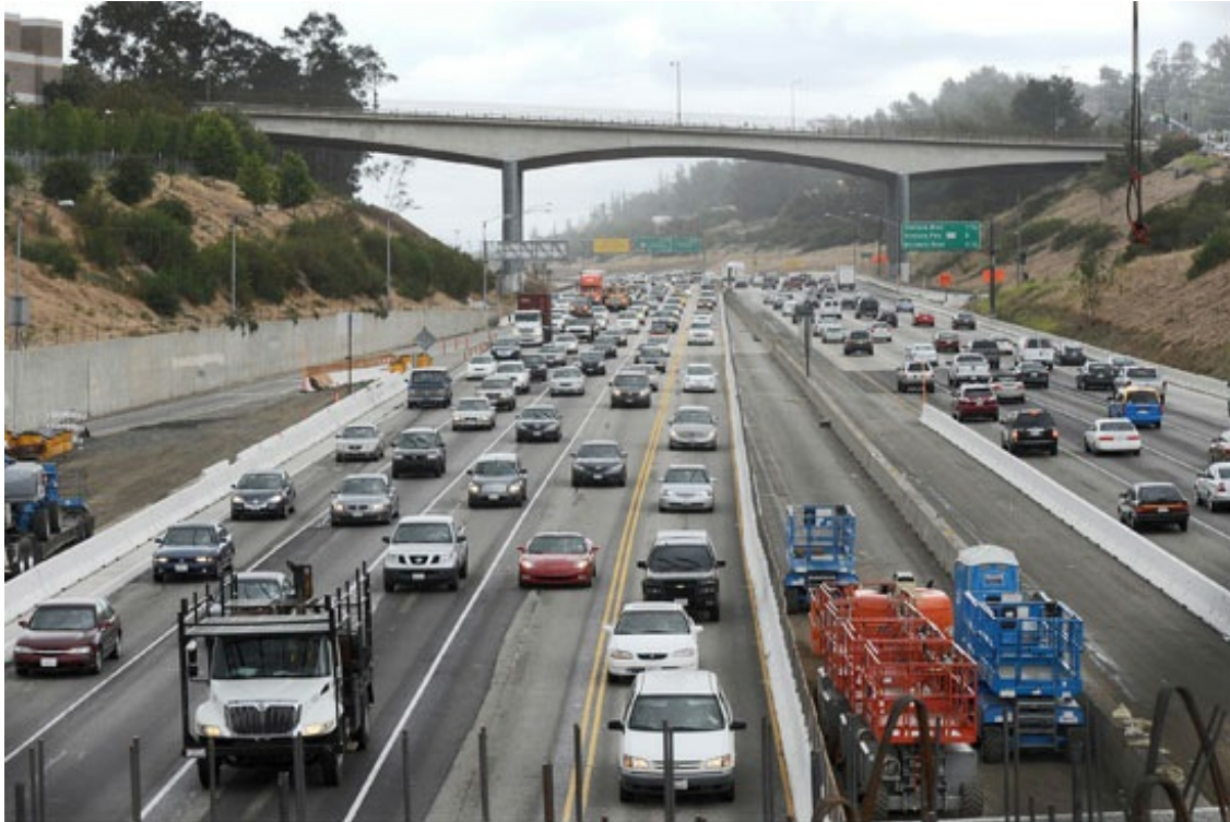
The Mulholland Bridge, looking north from access road near the 405.
