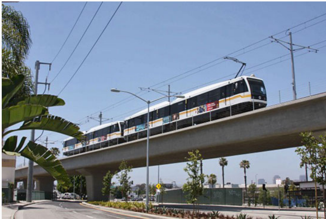
Expo trains are heading toward Culver City, with the station's opening set for June 20. Photo/Metro
