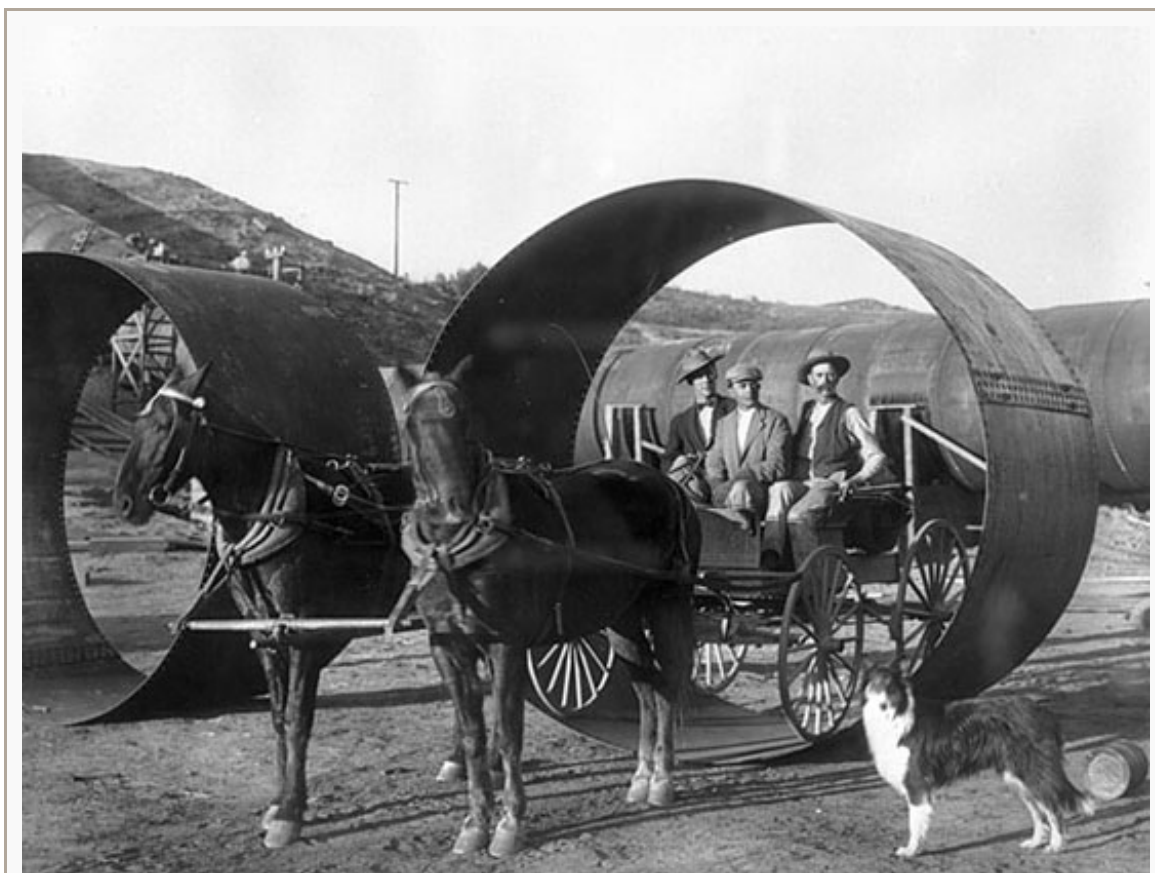
Undated DWP photo shows pipe used for aqueduct. Smaller pipe of the same riveted steel built the trunk line.
