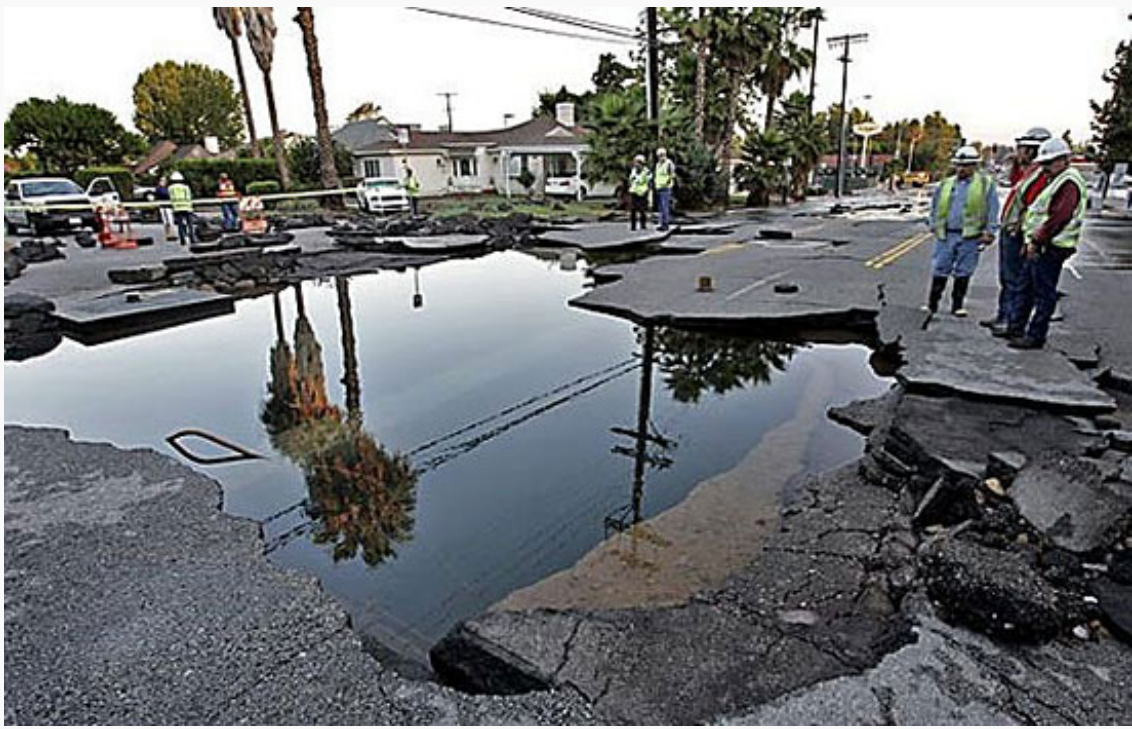
The 2009 rupture cost millions of dollars in damage. Photo/Los Angeles Times
