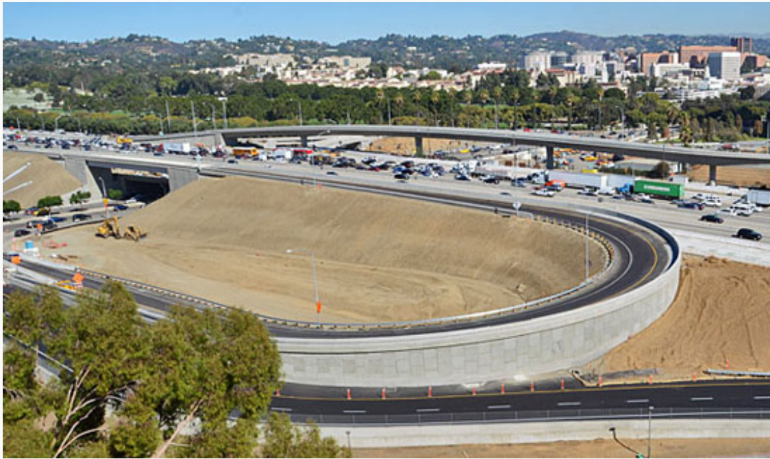
A view of the completed Wilshire interchange facing northeast, with the newest ramp in the foreground. All of the reconstructed ramps are open to the public as of Thursday. Photo/Metro
