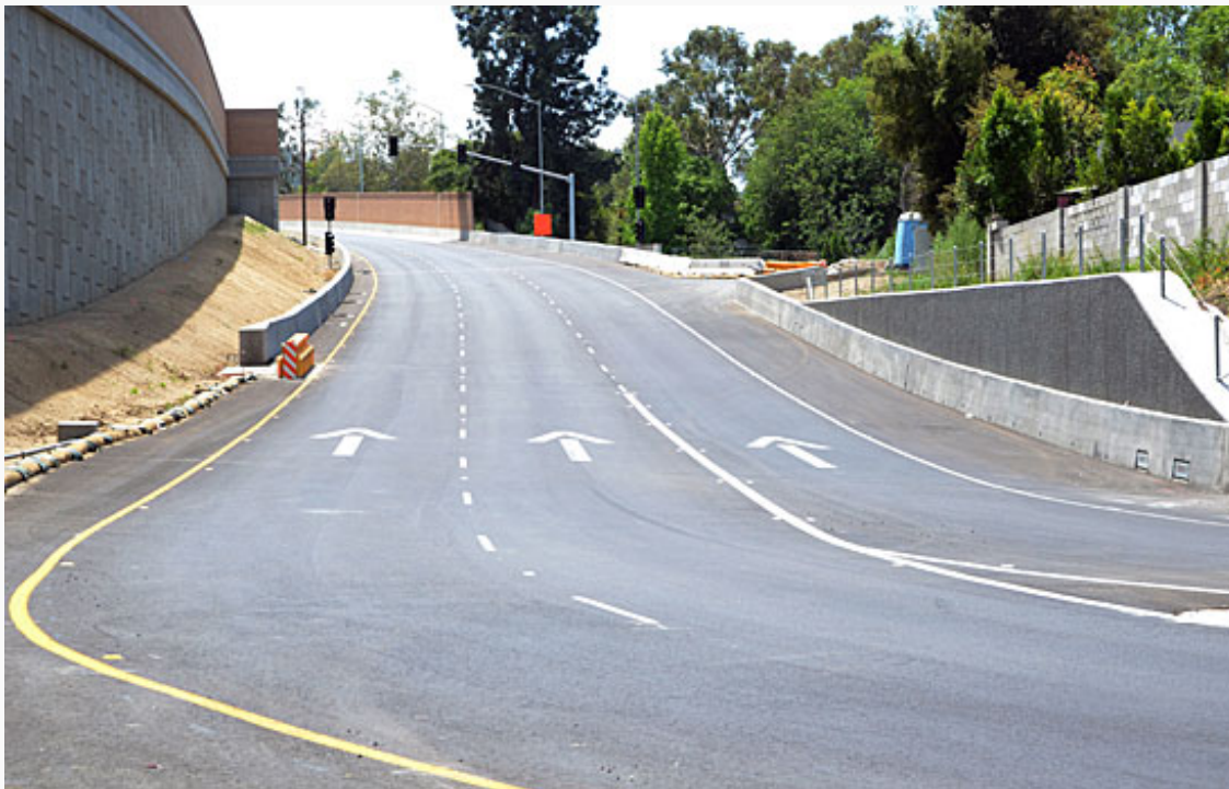
The Valley Vista on-ramp to the southbound freeway is 98% complete. Photo/Metro
