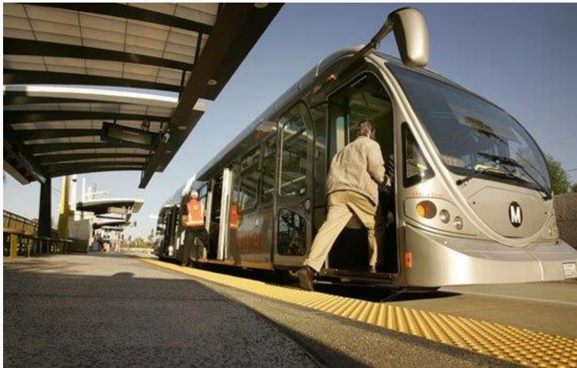
Gating the Orange Line's 18 stations is possible—for a price. Photo/Los Angeles Times
