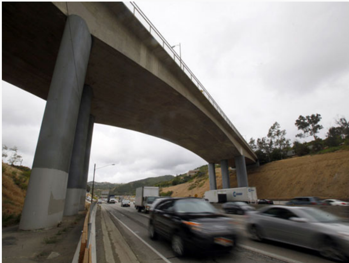
The Mulholland Bridge was demolished and rebuilt as part of the 405 Freeway improvements project.
