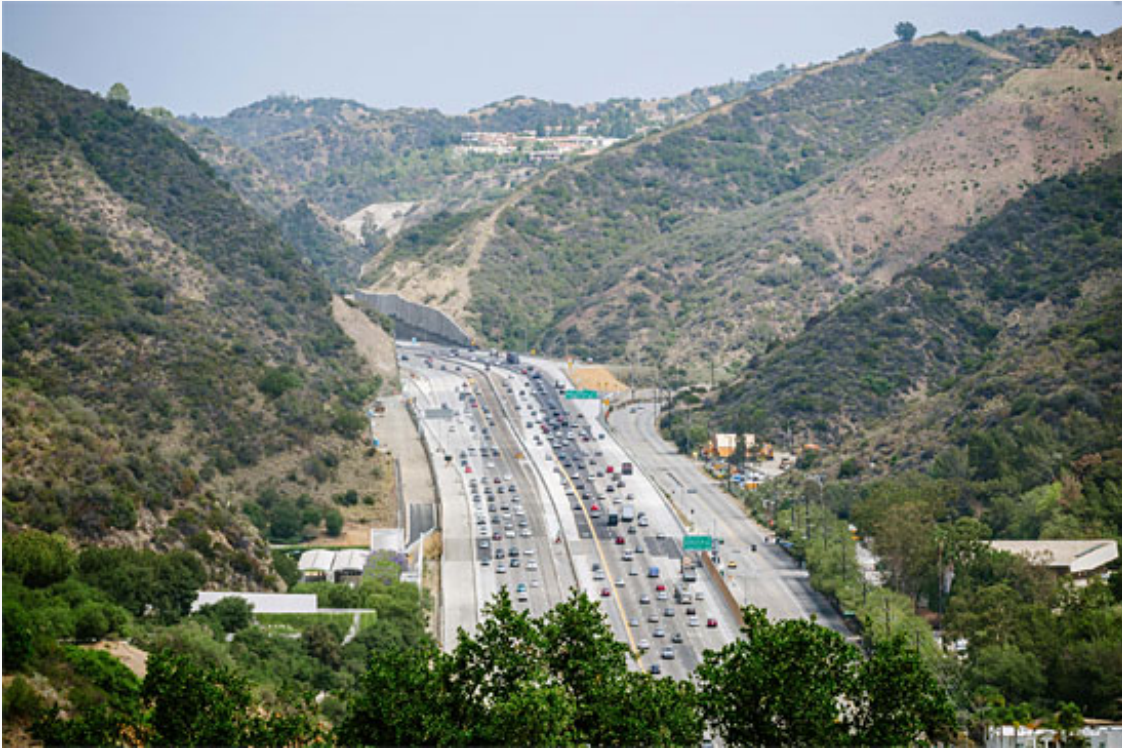
The bus line will roll through the Sepulveda Pass via the new carpool lanes. Photo/Metro's The Source
