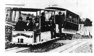
The Clay St. Hill Rallroad, San Francisco, California, was the first street cable car application: operations commenced in 1873. Andrew Hailidle, the inventor, is seated front center on the "gripper car" which towed the "trailer car" in both directions. Use of a separate car for locomotion was common practice in early street railway vehicles whether cable, steam, or electric.
