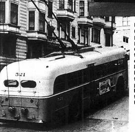
Electric rubber-tired trolley coaches (trackless trolleys) solved a common problem of many street railway companies which desired to remove deteriorated, expensive-to-maintain tracks while retaining inexpensive electricity to power vehicles. San Francisco Municipal Railway Coach No. 521 was delivered in 1947 by the St. Louis Car Co. during the peak period of trolley coach construction; between 1930 and 1952 over 8,000 trolley coaches were delivered to U.S. transit systems.
