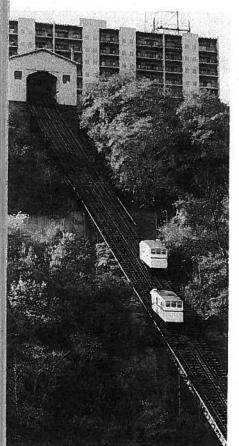
The Monongahela Inclined Plane, operated by the Port Authority of Allegheny County, dates from 1870. Two 3-compartment cars travel the 640 feet of track—set at a 38-degree angle against the side of Mt. Washington—In less than 2 minutes.
