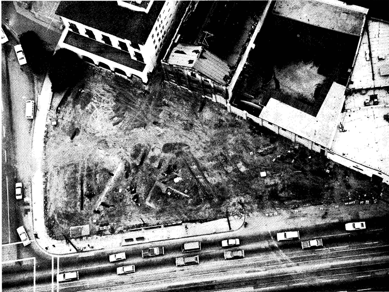
PLATE 8: La Placita Site Under Excavation. Alameda Street at bottom; North at right of photo. By John Shadle, City of Los Angeles, Department of Building and Safety.
