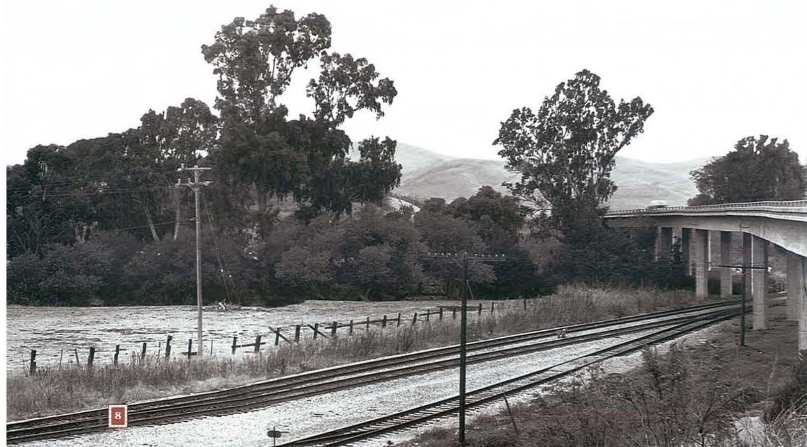
This site beneath a Highway 101 overpass was not proposed for the National Register.
