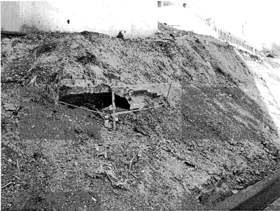
Figure 16. Exposed brick conduit near project area, east section
