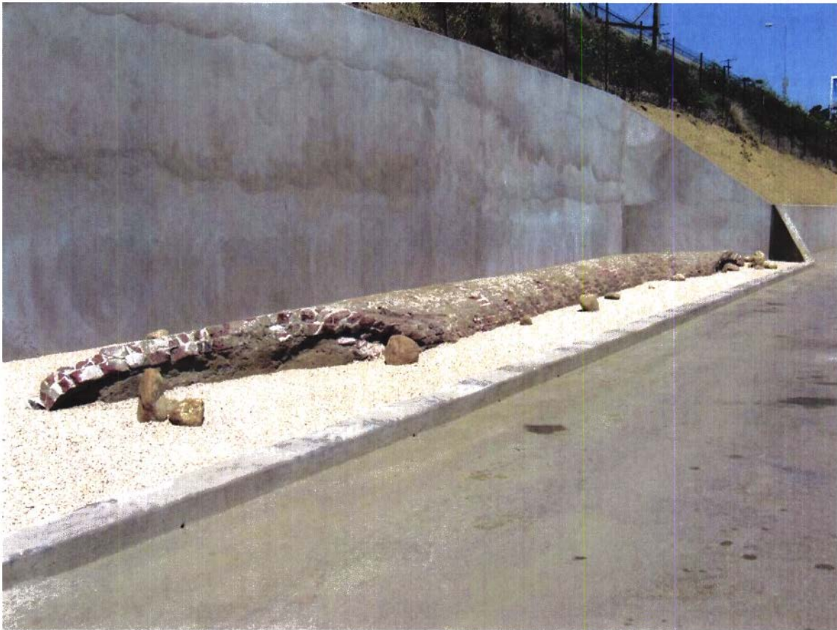
Figure 2.21. Zanja Madre final appearance, view to northwest
