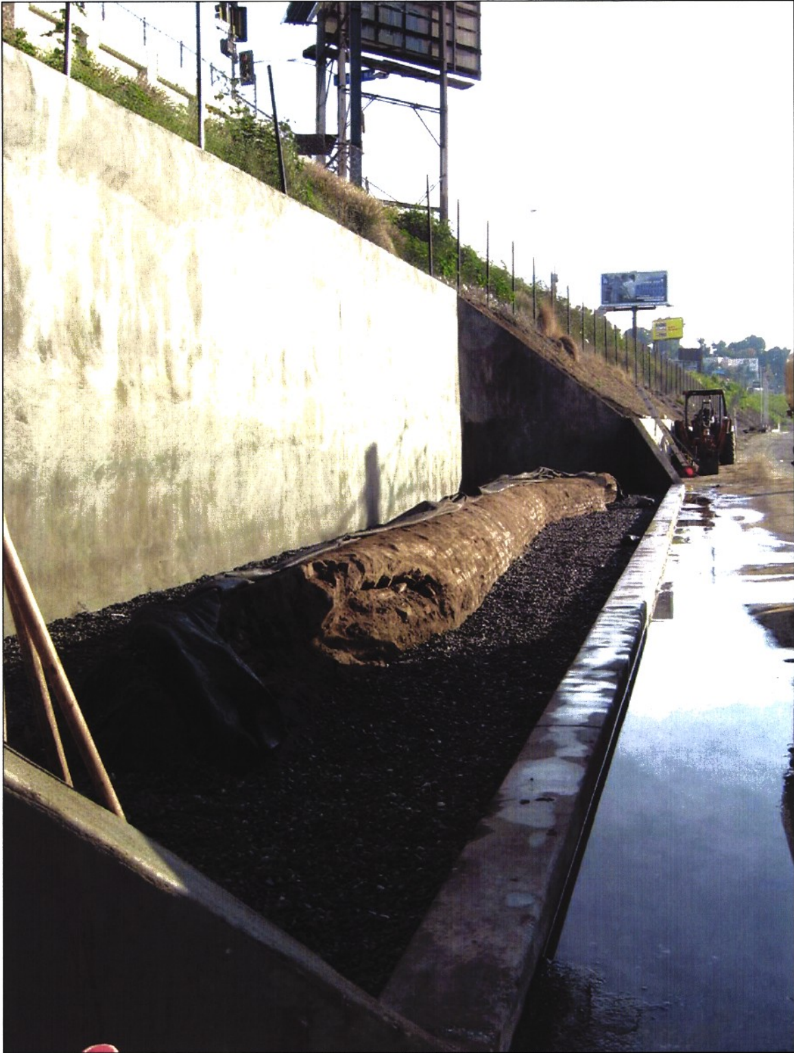
Figure 2.20. Zanja Madre with retaining wall & gravel, view to north
