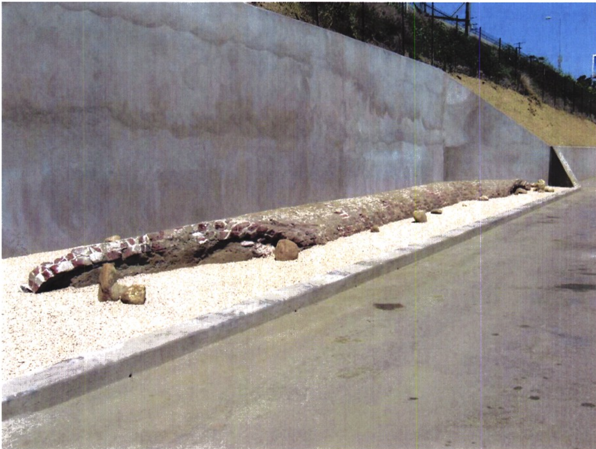
Figure 2.21. Zanja Madre final appearance, view to northwest
