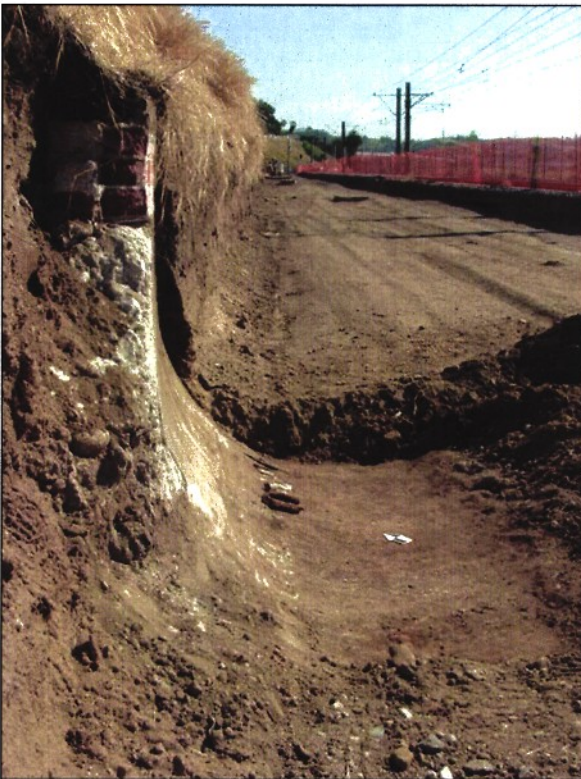
Figure 2.7. Feature 1, view to northwest, after clearing sediment
